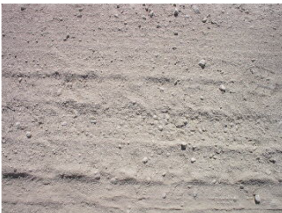
BEFORE STABILIZATION WITH TSB
