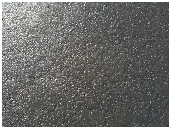
AFTER STABILIZATION WITH TSB
