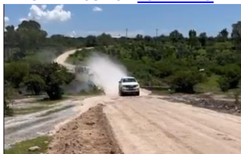
BEFORE DUST CONTROL WITH TSW
